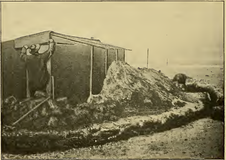
BUILDING THE STORE HOUSE. GJÖAHAVN, 1903.
